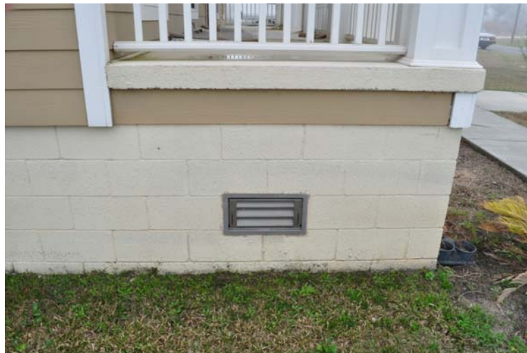
Fig. 2.2. PHOTO: Flood vent in foundation wall.
